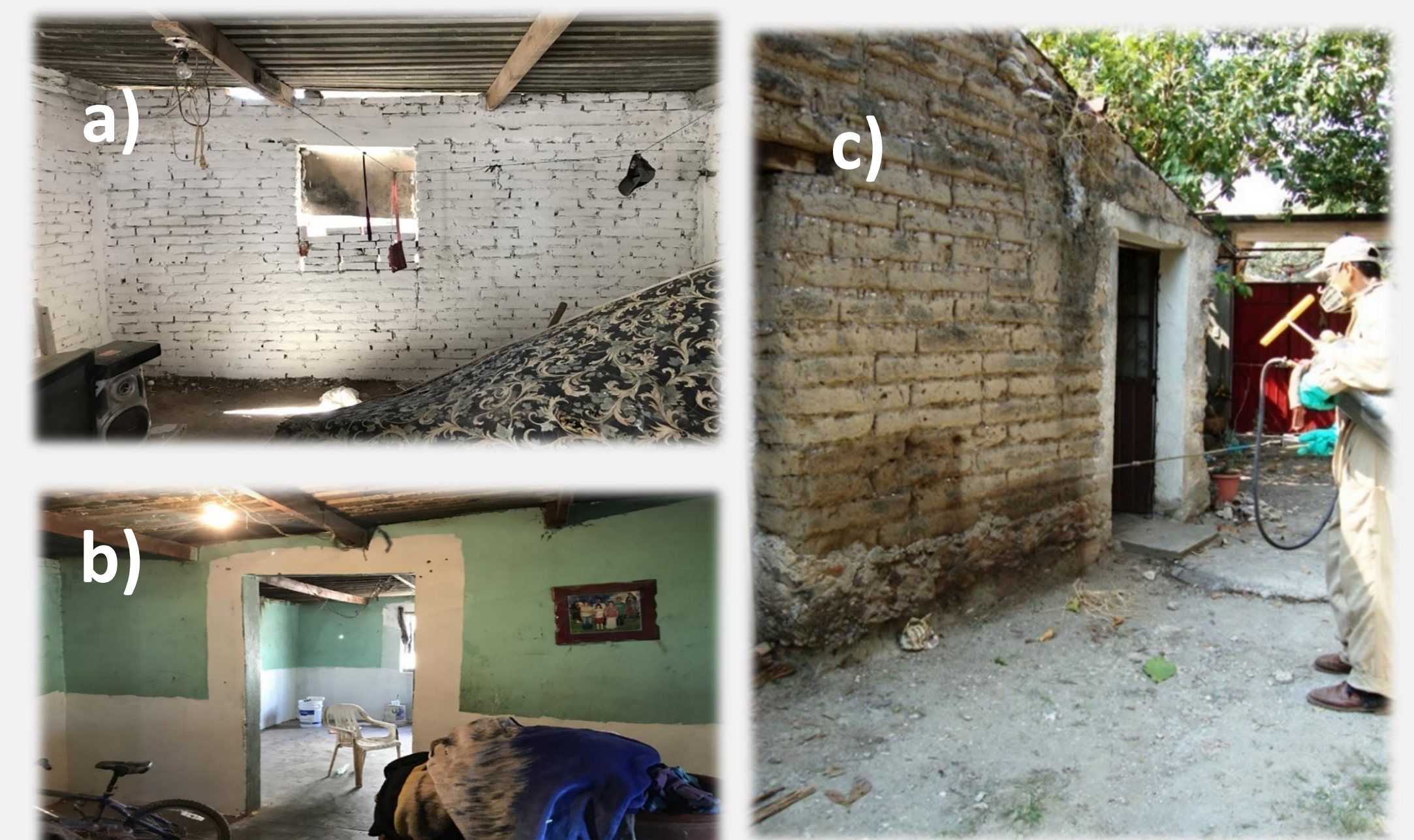
Fig. 4 Treatments: a) total painting of walls, b) painting up to 1m to floor level and c) residual spraying.
