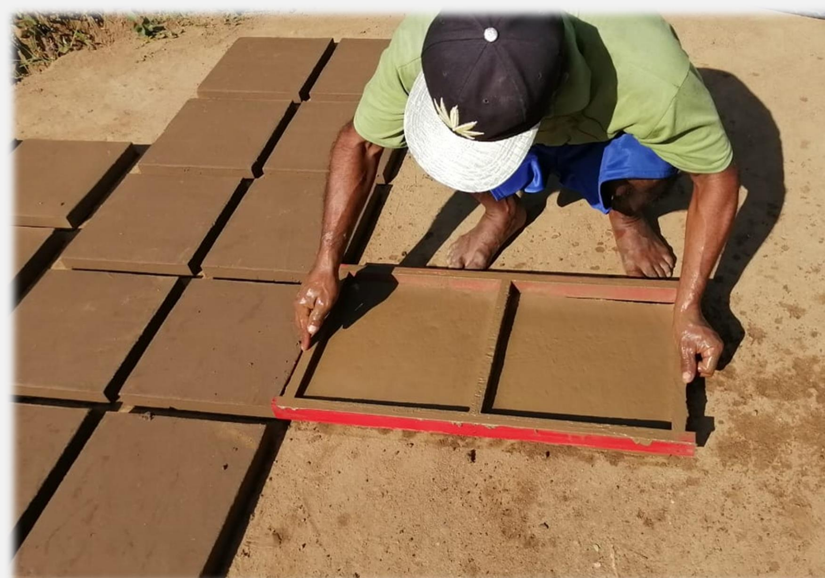
Fig. 1 Elaboration of bajareque (mud) substrates in Pochutla, Oaxaca, Mexico.
